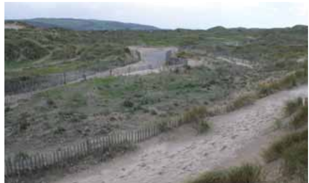
Fencing to control erosion of sand dunes. Control of public access can prevent damage to sensitive habitats and help reptiles to survive in areas otherwise subject to high visitor pressure (Helen Demopoulos)
